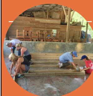
Learning to frame walls for a new church in Roatan
